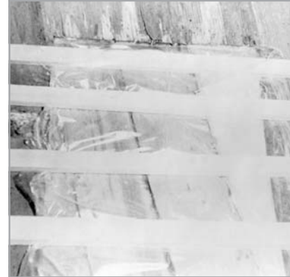
Figure 5-17 Cover the stringers with plastic to prevent bonding. (View from inside of hull).
