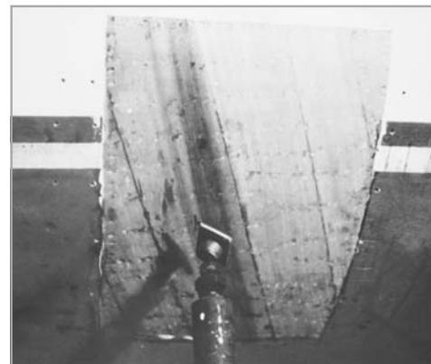
Figure 5-19 Continue until all the layers are completed, matching the skin thickness.
